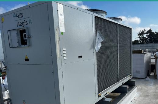
backup heating. Not only does Aegis operate at lower ambient temperatures than many alternative solutions, but it also maintains the ability to deliver hot water well above 140°F when the weather turns colder. CO<sub>2</sub> refrigerant also exceeds expectations when compared to other common refrigerants used in heat pump water heaters with a Global Warming Potential (GWP) of 1.
